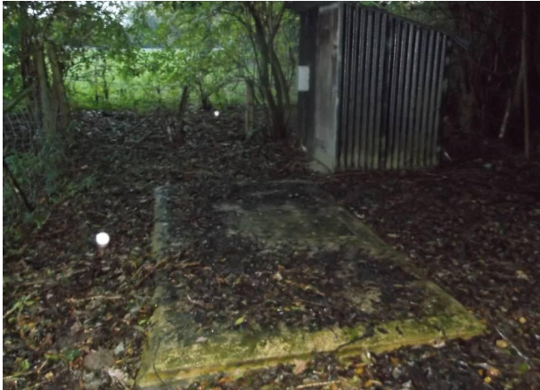
Figure 22: Situation of tank
