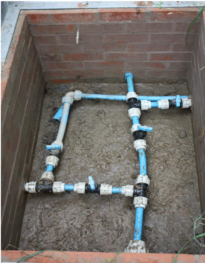
Figure 25: Valve chamber
