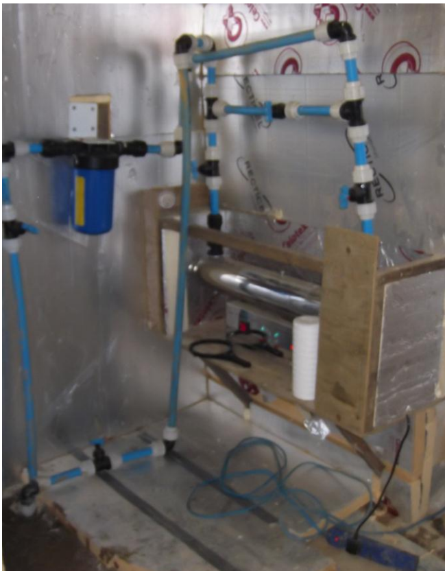
Figure 21: Treatment arrangements showing filter and UV tube
