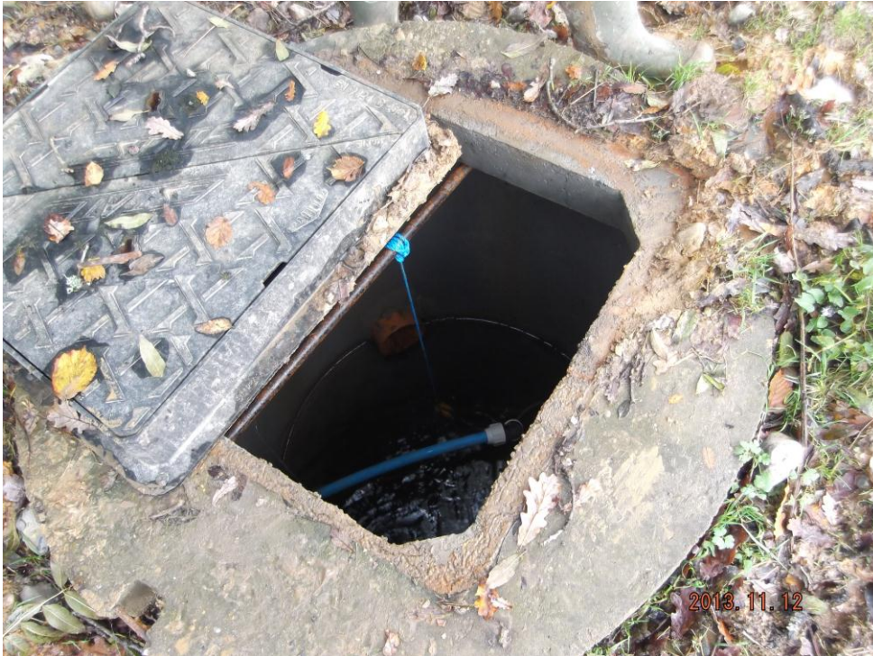
Figure 20: Spring collection chamber
