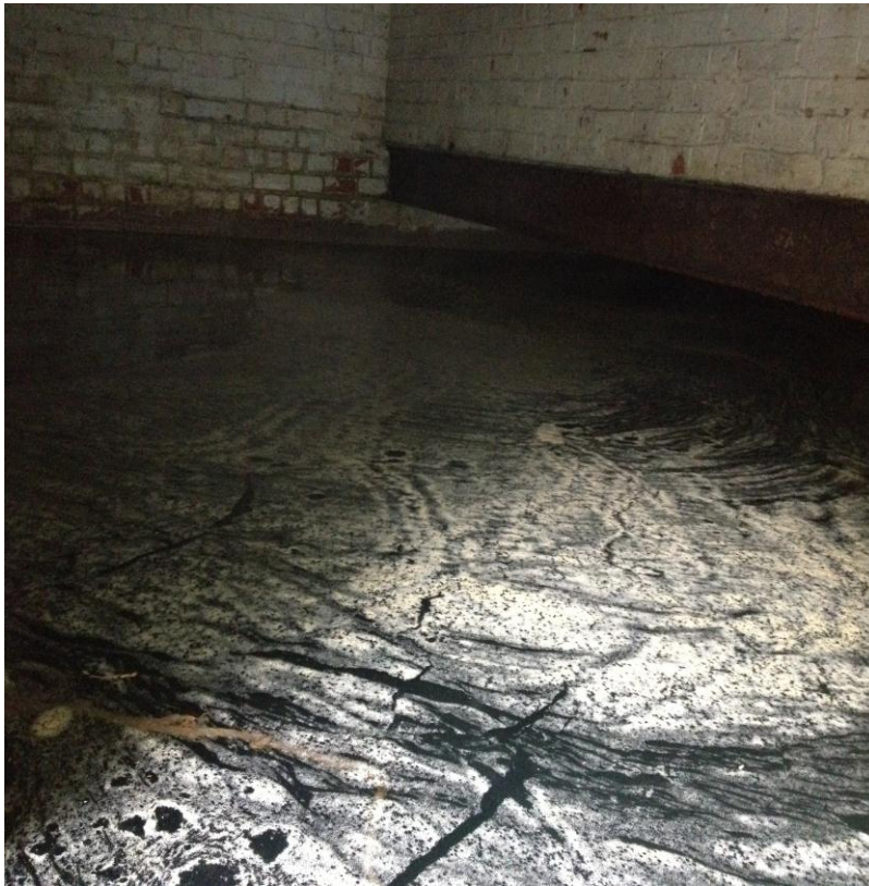
Figure 12: Leachate floating on the water surface
