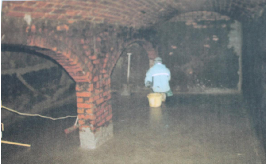
Figure 24: Cleaning inside the vaulted brick reservoir
