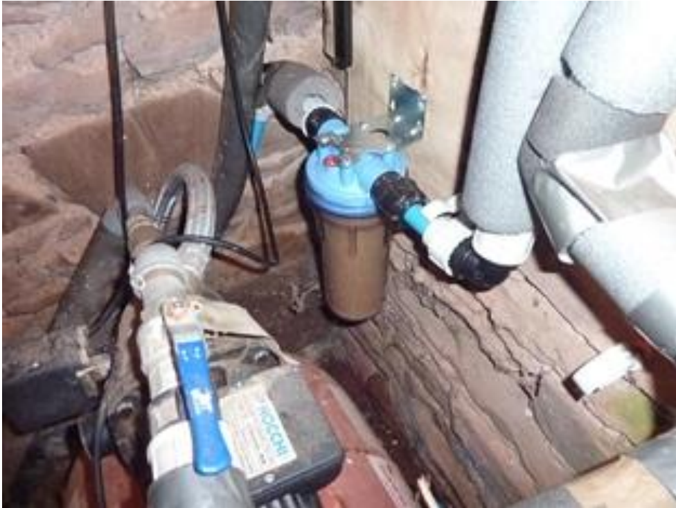
Figure 16: New 5 micron cartridge filter prior to UV disinfection
