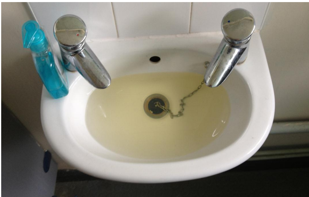
Figure 14: Discoloured water at a handbasin
