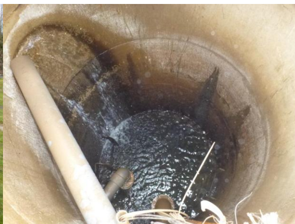
Figure 19: Old Well interior showing iron-ductile pipework rising main, incoming raw water supply from South West Water
