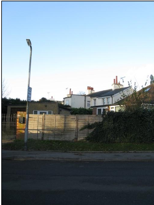
Figure 26 - A view of the rear of 95-97 High Road, showing the attractive nature of the high chimney pots on this row of houses.
