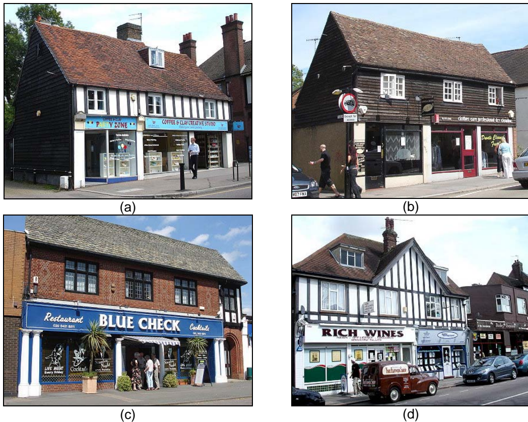
Figure 28. Character Zone 2: negative factors; examples of modern shop fronts inserted into older style properties on the High Street. Nos. 46 – 48 (a); 56 & 58 (b); 144 – 146 (c); 110 – 118 (d)
