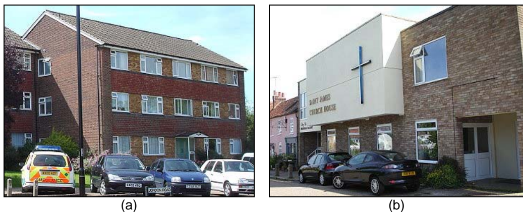
Figure 21. Character Zone 1: negative impact; Grove House (a) and Church House (b), High Street
