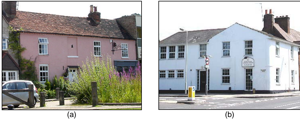
Figure 20. Character Zone 1: loss of traditional architectural features; replaced doors and windows in the High Street, Prospect Cottage (a) and No. 2 (b)
