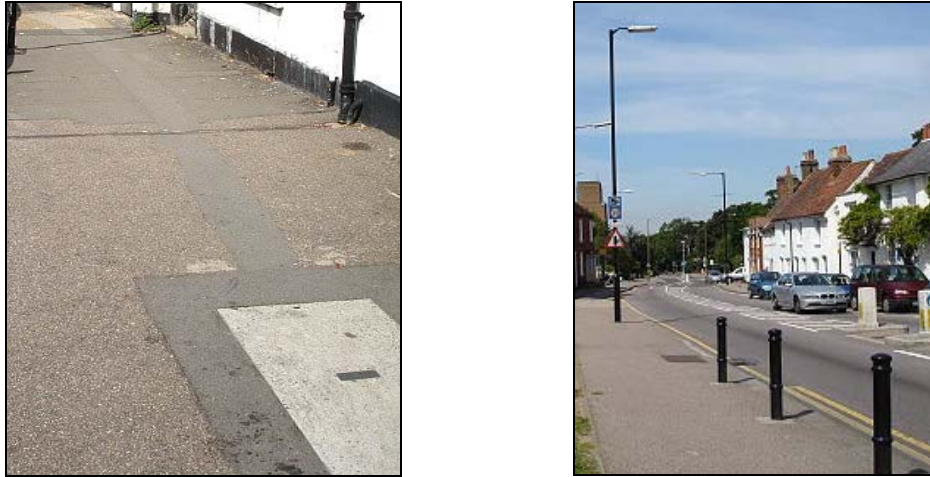
Figure 18. Character Zone 1: negative factors; poor street paving, the use of bollards, and tall lamp posts on the High Street
