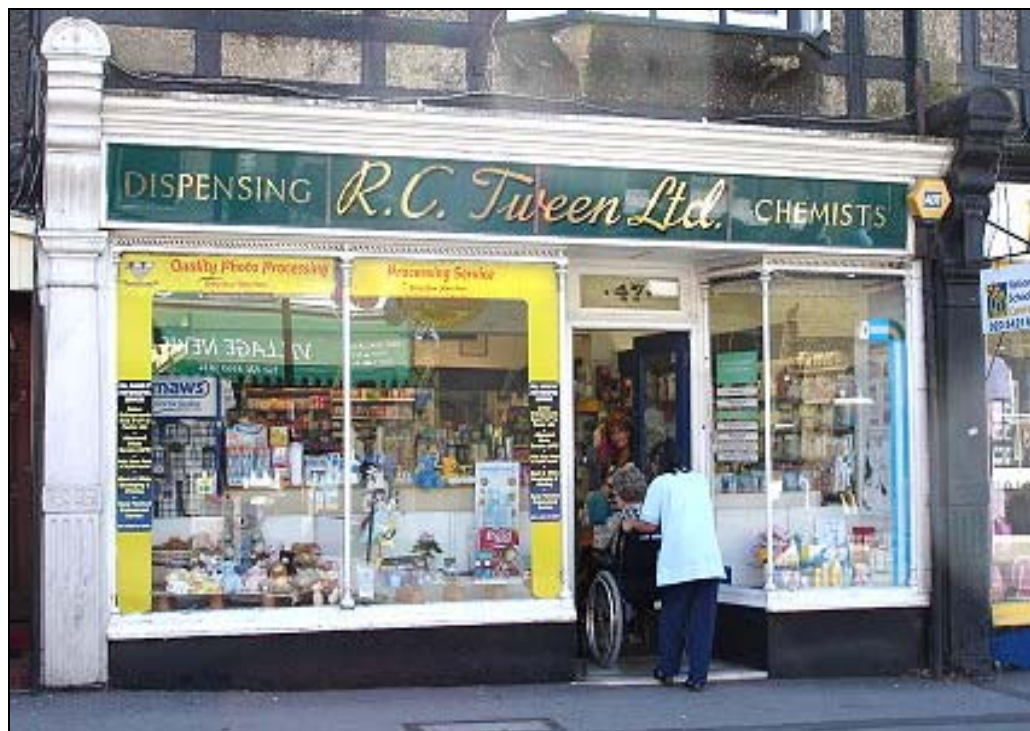
Figure 29. Character Zone 2: a good example of a retained shop front with large display windows, traditional hand painted fascia, pilasters, consoles, stall riser and a recessed doorway with fanlight over (47 High Street)
