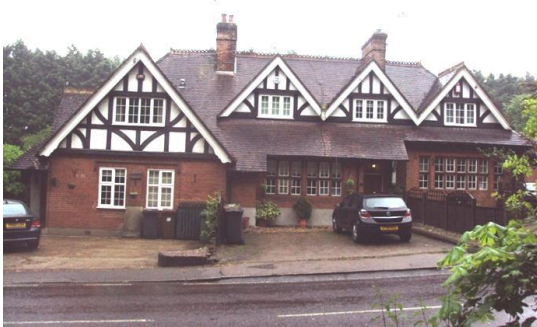
Figure 2: 5-9 Elstree Hill North (Left)
