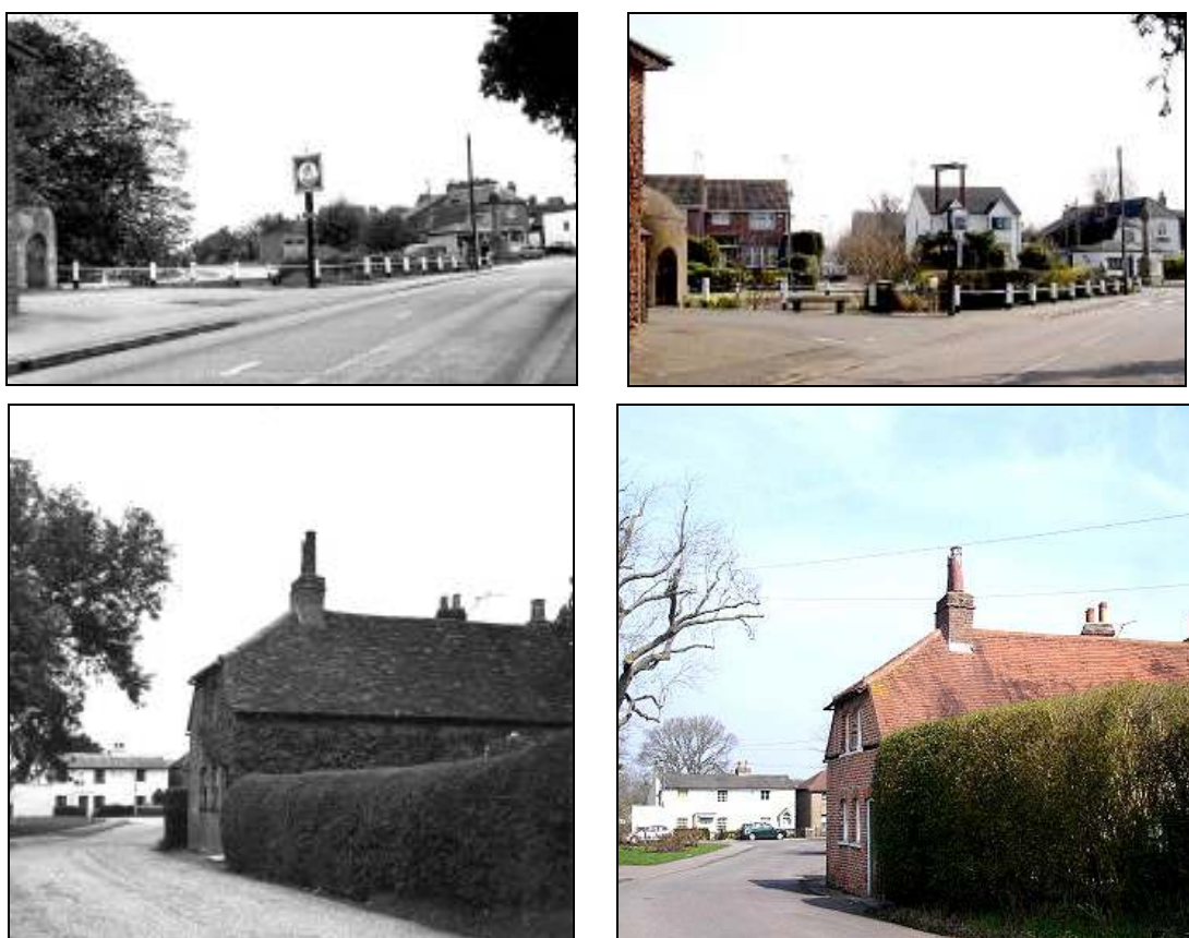
Figure 5. 1969 and 2011. Above: towards the pond. Below: Pound Lane.
