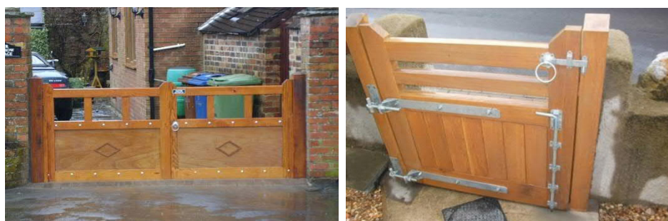
Figure 5-4 Example of flood gates
