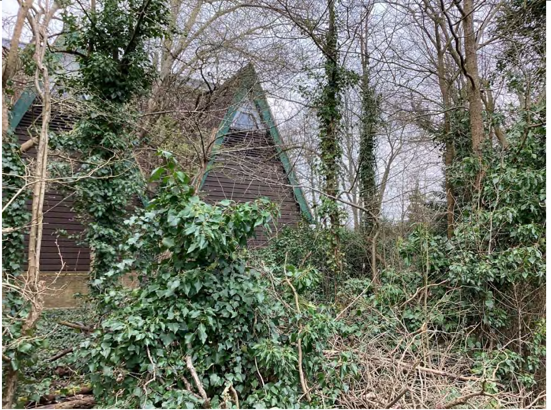
Photograph 3: View of SA-82 from Public Right of Way, showing north-east corner with boundary vegetation and a sports centre building belonging to the school campus.
