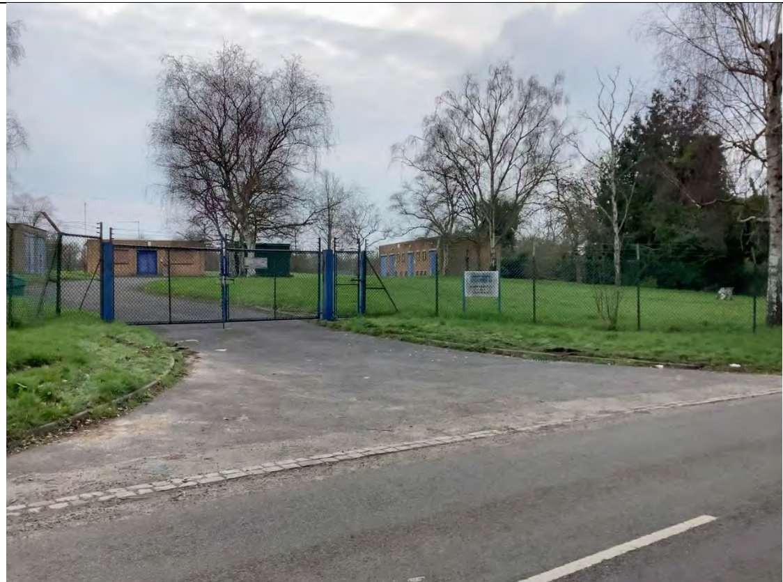
Photograph 4: View of facing south-west from Berry Grove Lane, showing view of utility sub-station.
