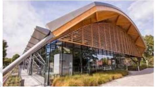
Figure 3.7: The WWF Living Planet Centre, Woking, uses double instead of triple glazing as it was more carbon efficient over the lifetime of the building.
