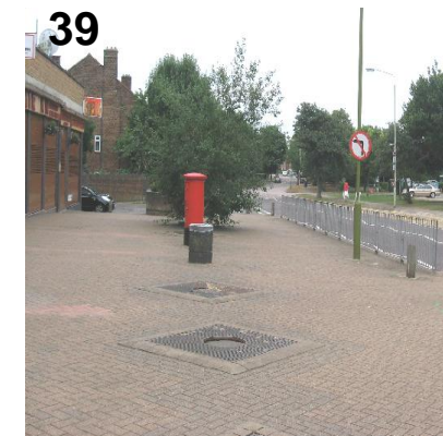
36. Note how the pattern has been laid incorrectly (top left).
