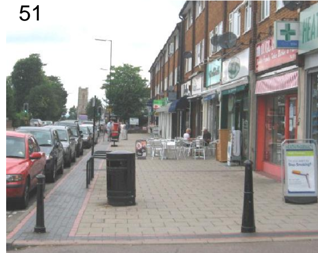
51. Note the well-placed street furniture, although the bin in the foreground could have been placed a little more to the left.
