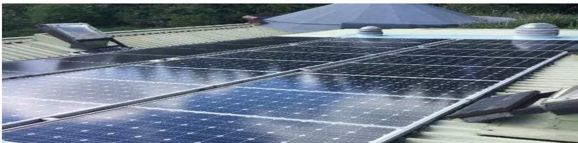
Figure 17: Solar panels installed on the roof which is used for rainwater collection.
