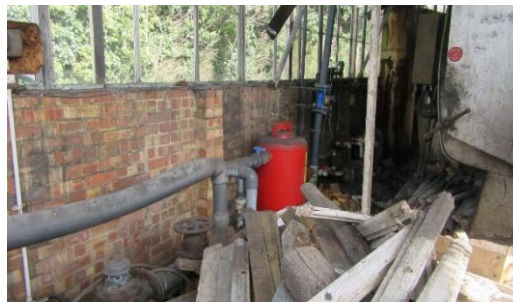
Figure 21: Supply pipework in an inadequate and unacceptable environment
