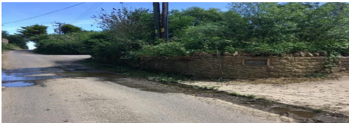
Figure 28: Leak on the old supply
