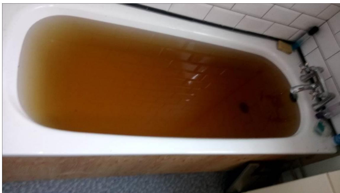
Figure 23: Extent of discolouration of water
