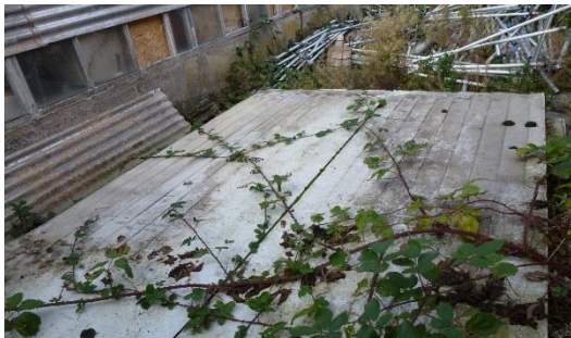
Figure 20 : Vegetation covering poorly constructed well cover
