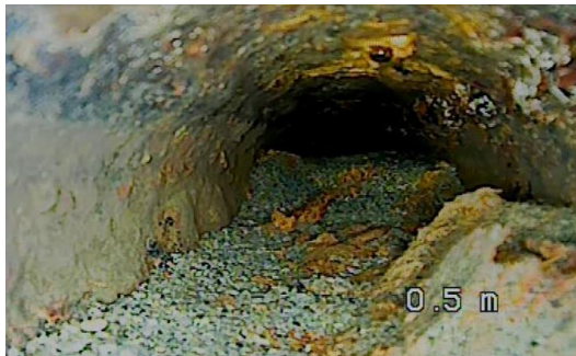
Figure 26: Sediment in pipework
