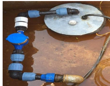
Figure 27: Poorly constructed headworks on source
