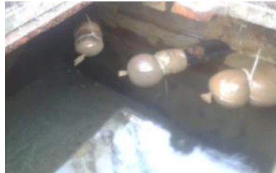
Figure 25: Tights being used as filters in a collection chamber
