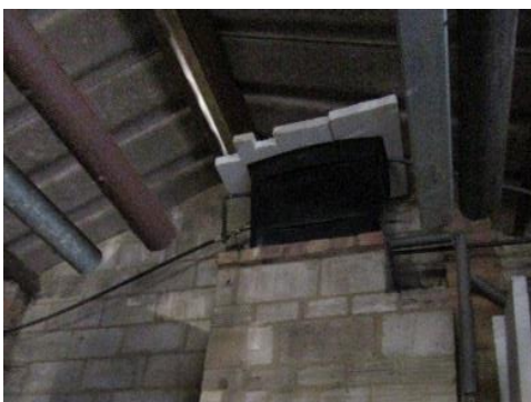
Figure 22: Header tank with overlaid polystyrene strips as a cover
