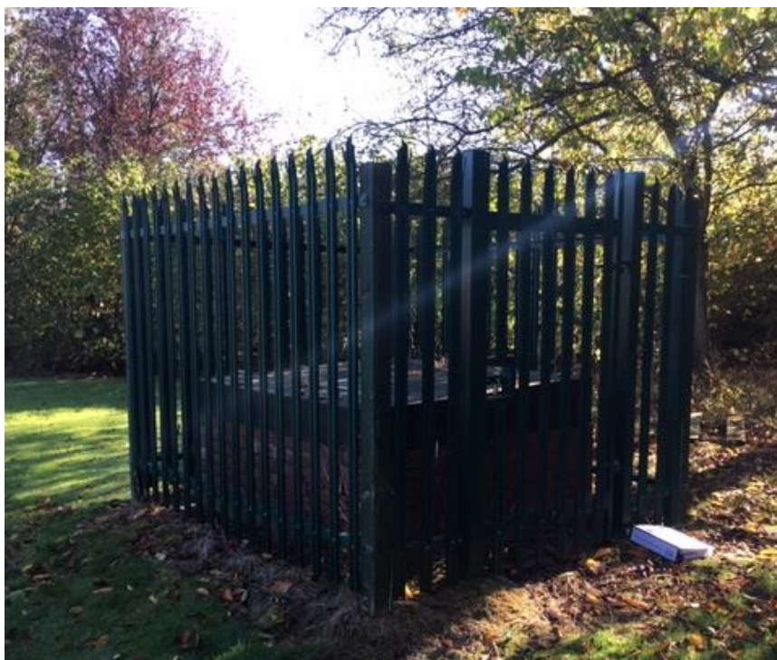
Figure 29: Robust source protection on a private supply to a hospital
