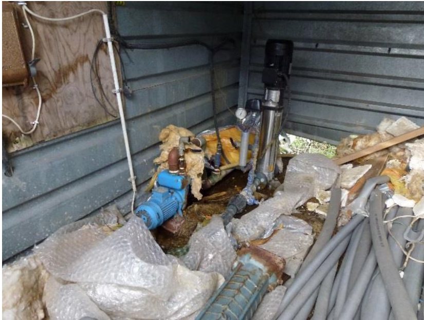
Figure 18: Distribution pipework before major corrective work
