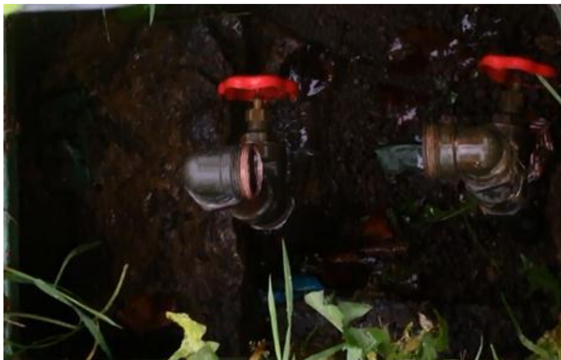
Figure 20: Pipework after illegal cross connection had been removed
