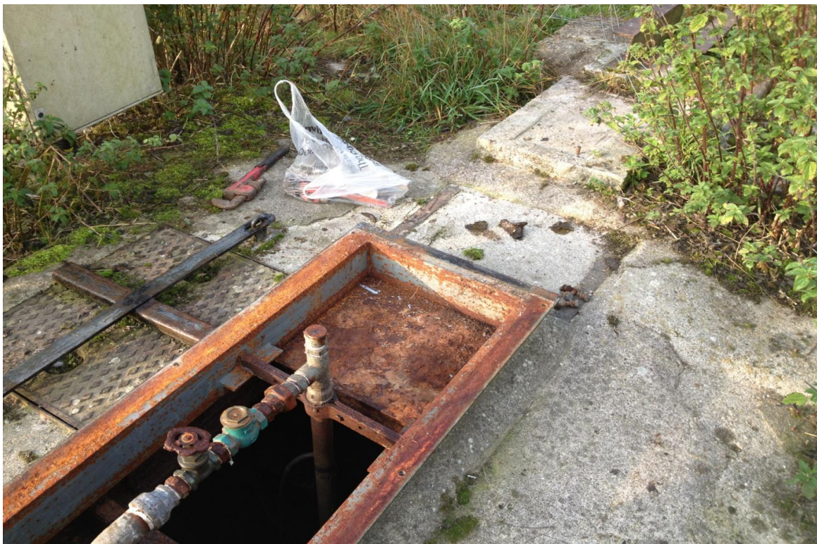
Figure 18: Area directly around borehole
