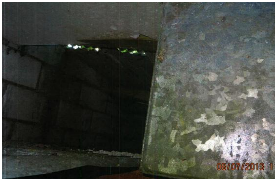
Figure 19: Storage tank with holes in roof
