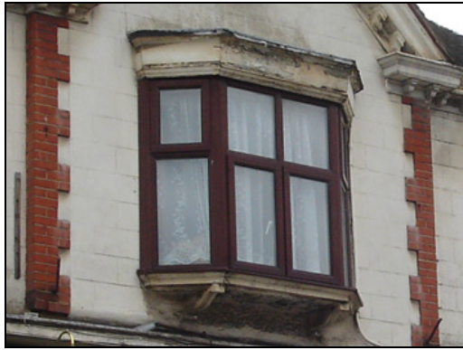
Figure 21. Character Zone 1: loss of traditional architectural features; replaced windows in the High Street
