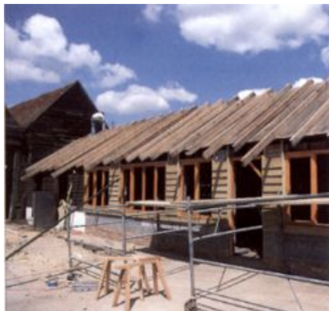
Conversion of farm building
