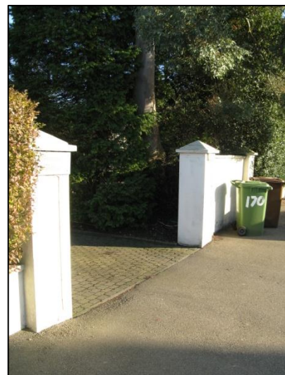
Figure 21 - Attractive entrance gateposts to 170 and 172 High Road.
