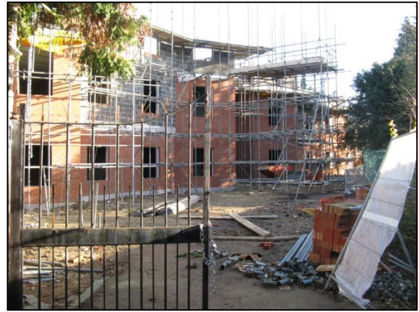
Figure 17 - The development of flats under construction, viewed from the Windmill Lane side.
