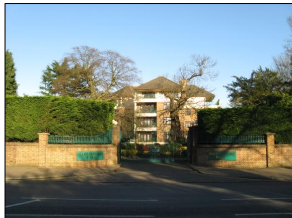
Figure 31 - The main entrance of Hartsbourne Park
