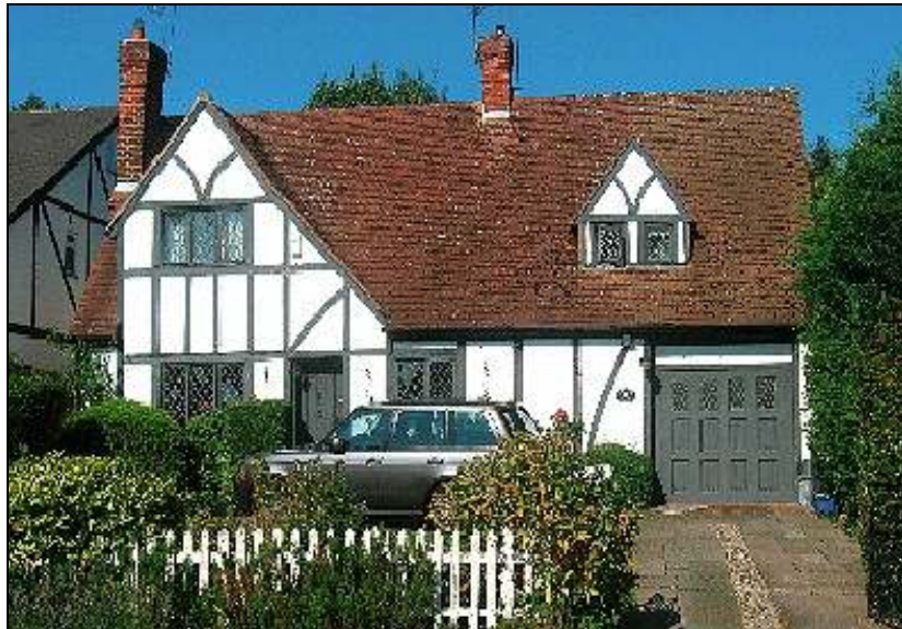
1 Mountway: an original 1920s house
