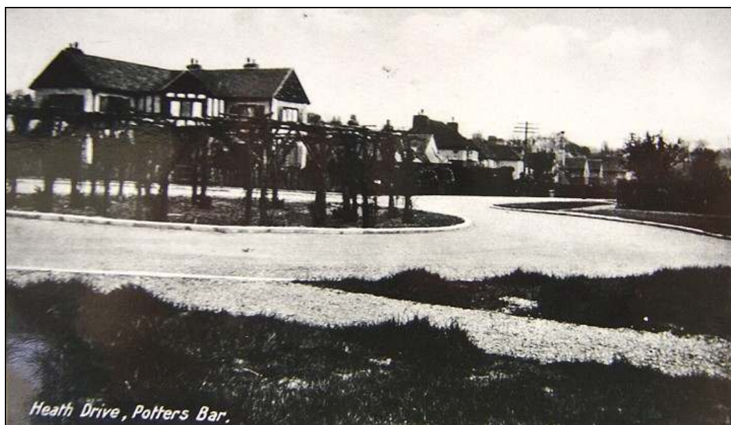
Heath Drive taken by the island at the junction with Manor Way soon after the new houses were built (HALS Photographic Collection: 78B4a). Thought to date to c1930 and, like the photograph above, it shows the beginnings of the Potters Bar Garden Estate with its tree lined road, grass verges, hedges, pavements and detached houses.
