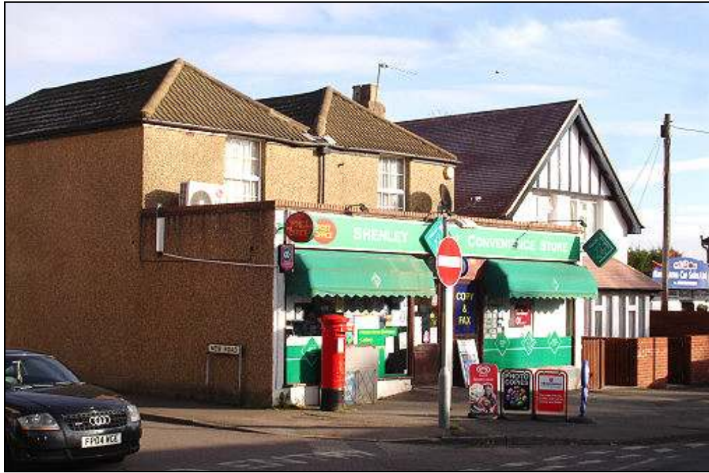
Figure 13. Unattractive shop front
