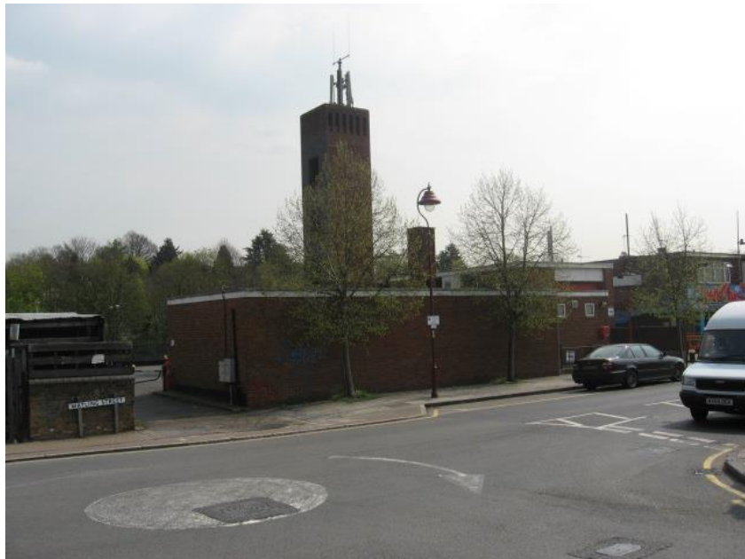
Photograph 2: The former Radlett Fire Station viewed from the west
