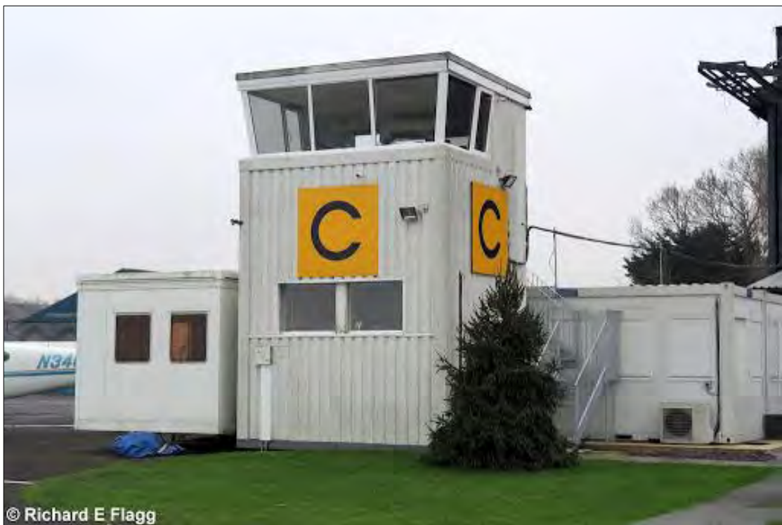
Figure 9 – ATC Tower at Elstree Aerodrome
