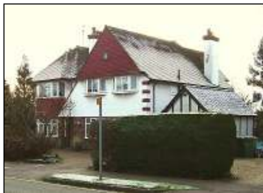
36 Heath Drive; an original 1920s house
