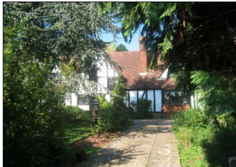
'Tudor', 5 Mountway: an original 1920s house
