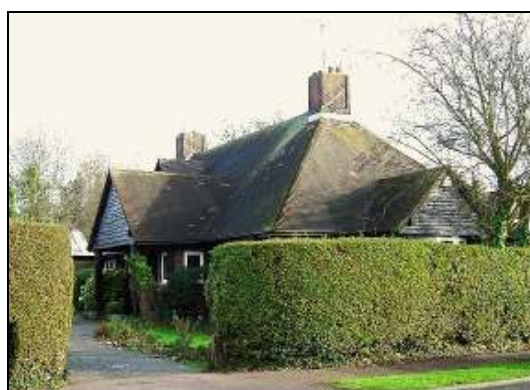
45 Heath Drive; an original 1920s house
