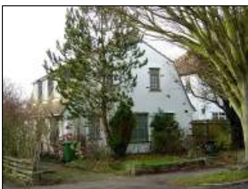
44 Heath Drive; an original 1930s house
