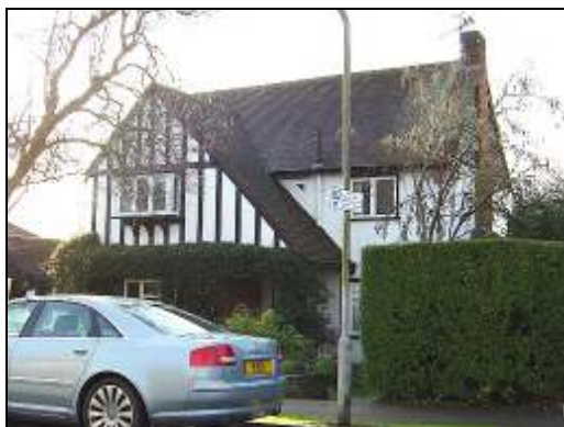
24 Heath Drive; an original 1920s house
