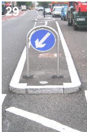
29. Hoop mounted keep left signs are preferred due to the sleek and visually simple appearance. (Image taken from the English Heritage publication 'Streets for all-East of England') / Manual for Streets.
