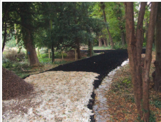
Use of a Cellular Confinement System to allow access for construction traffic through retained trees.
