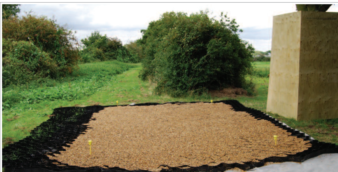
Ground protection used effectively to allow for construction within a tree root protection area, and the tree stem appropriately protected from any collision with construction vehicles.
