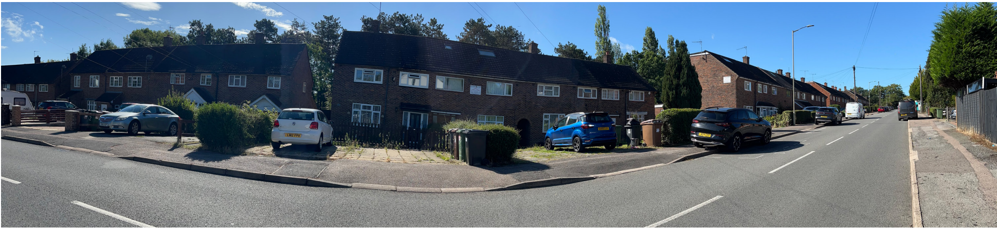
Fig 116. Residential street with street planting compromised by on-plot parking
