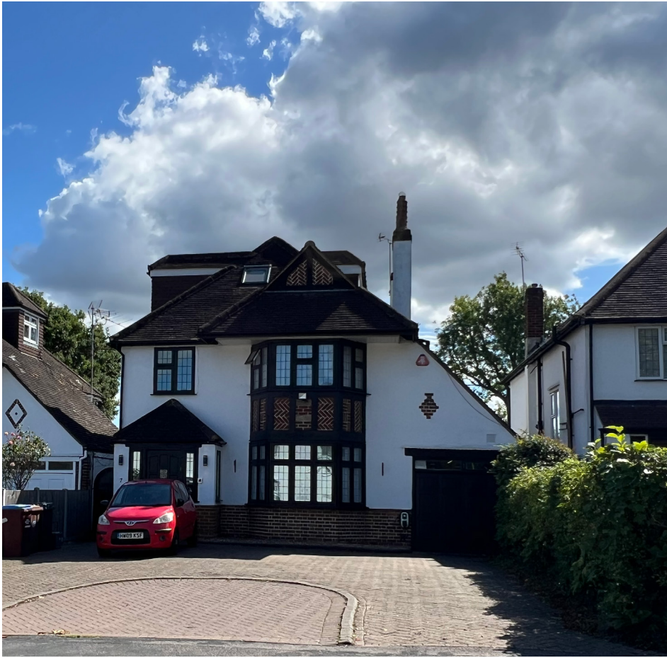
Fig 128. Interwar period rendered houses with decorative details on the bay windows.
