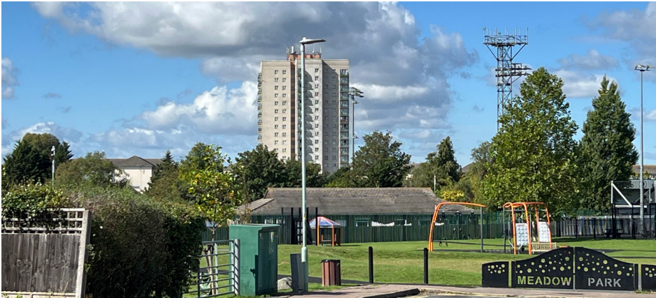
Fig 87. Canterbury House view from across Meadow Park
