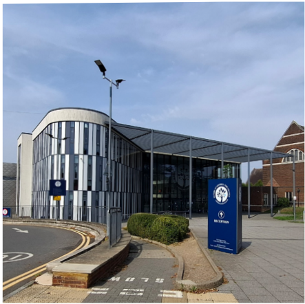
Fig 115. New school building
