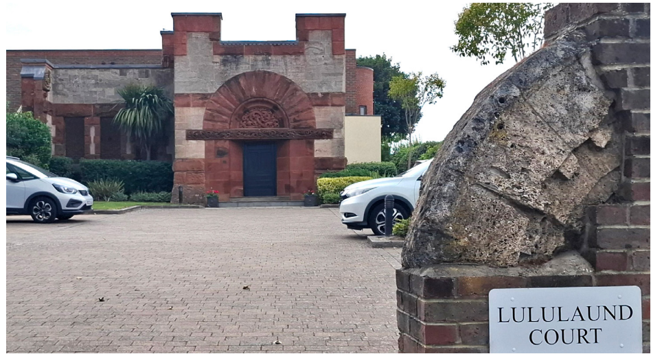
Fig 167. Fragment of Lululaund, Grade II*, completed 1894 for Sir Hubert von Herkomer, with elevations designed by H.H.Richardson.
