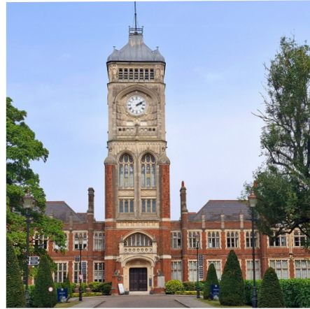
Fig 114. A former school conversion.
