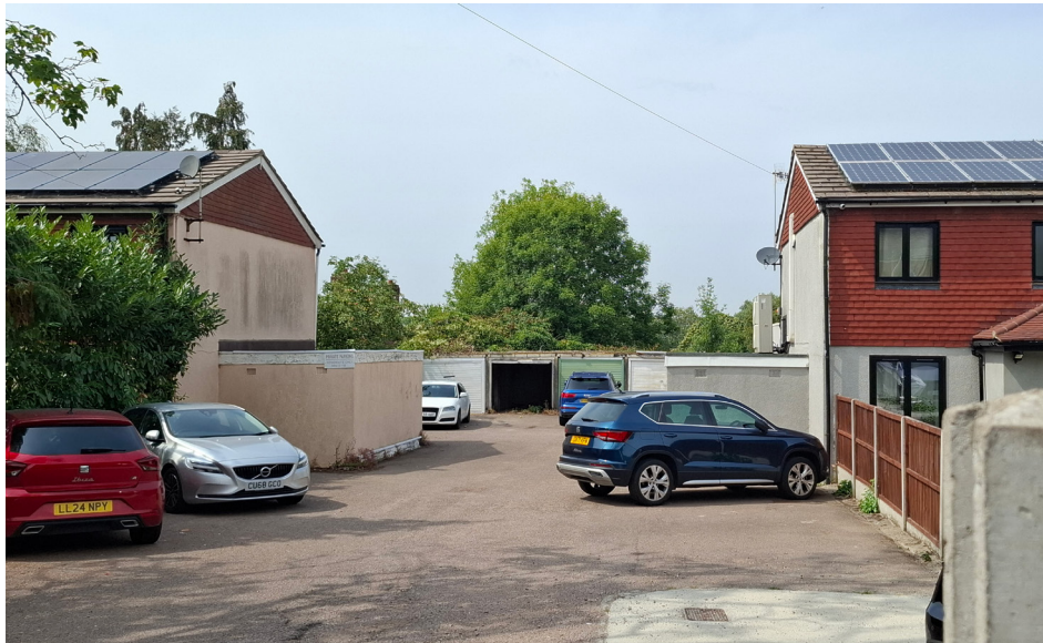
Fig 74. The prevalence of car ownership has sometimes resulted in a concrete-dominated streetscape.
