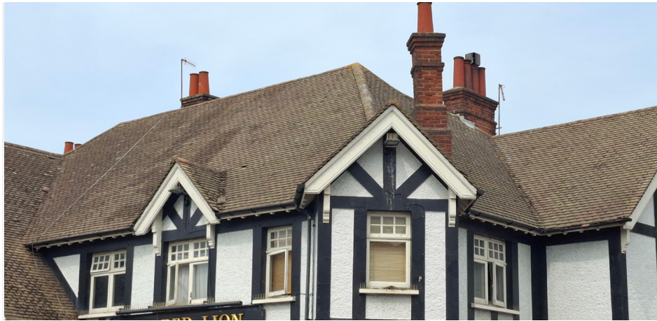
Fig 151. Mock half-timbered structure
