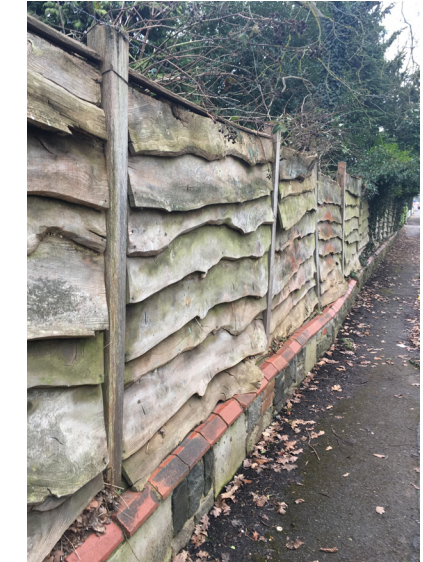
Untreated Weatherboarding Fence atop low brick wall
