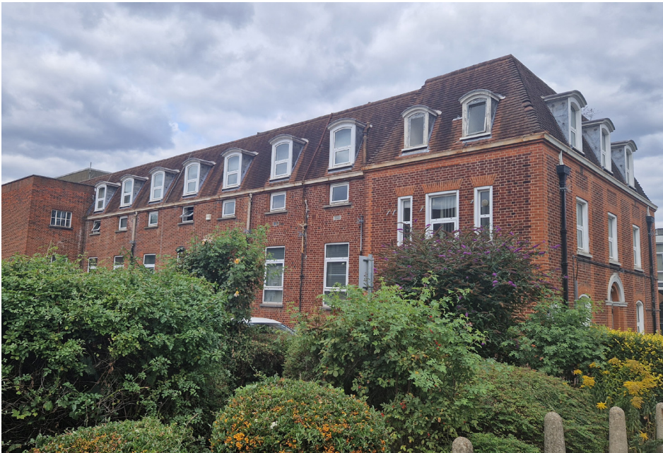
Fig 122. The Telephone Exchange building on Hatfield Road is currently vacant and a potential significant asset in Potters Bar
