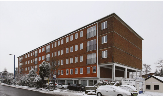
Fig 167. 230 High Street, Hollies House – Available
