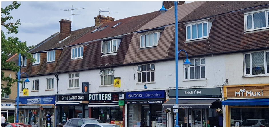
Fig 87. Town Centre terrace on Darkes Lane with active ground floor
