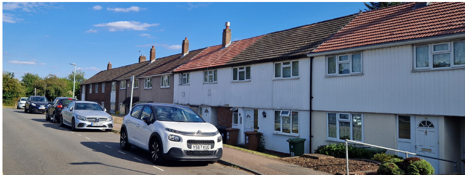
Fig 86. Terraced housing on Mutton Lane
