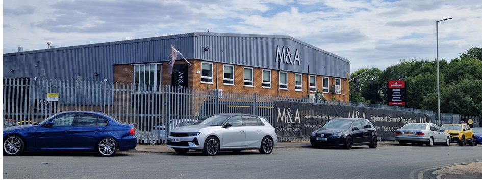
Fig 88. Large footprint industrial building
