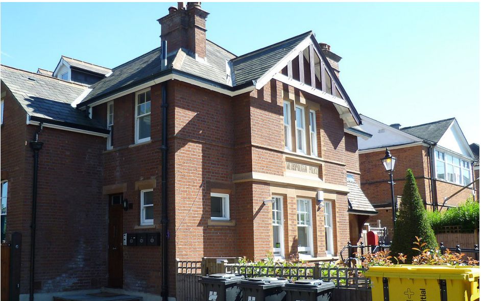
Fig 126. The Causeway Former Police station
