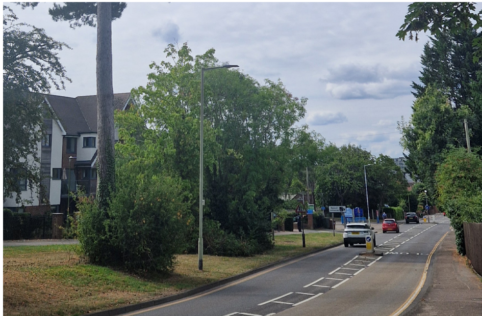
Fig 93. Through Route / Arterial Road Street Character – Darkes Lane near Little Heath
