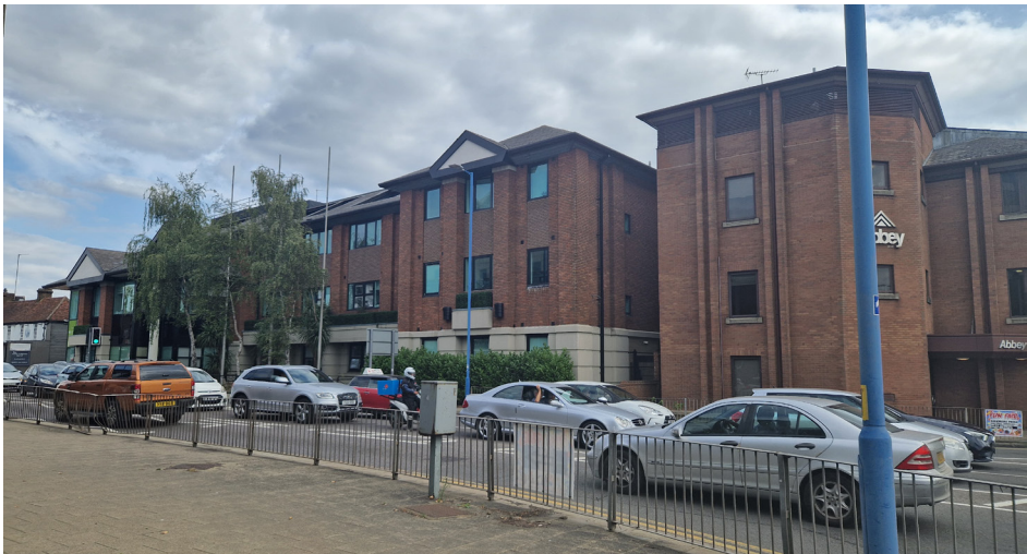
Fig 70. Converted residential building at junction between High Street and Mutton Lane
