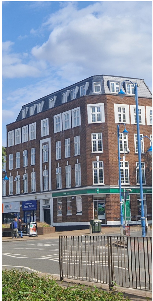
Fig 84. High rise office building on Darkes Lane
