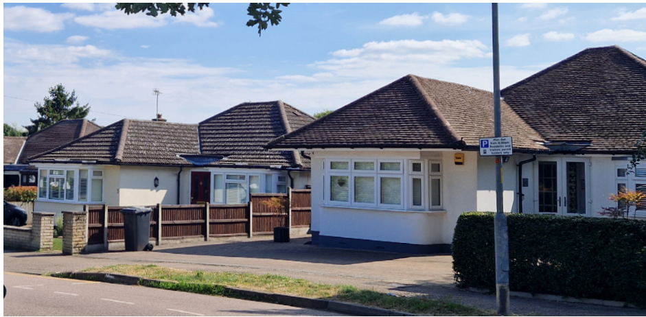
Fig 82. Detached houses on Daleside Drive
