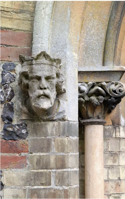
Fig 124. Decorative masonry details
