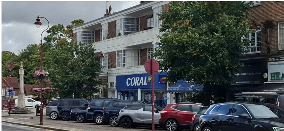
Fig 93. Flats over retails
