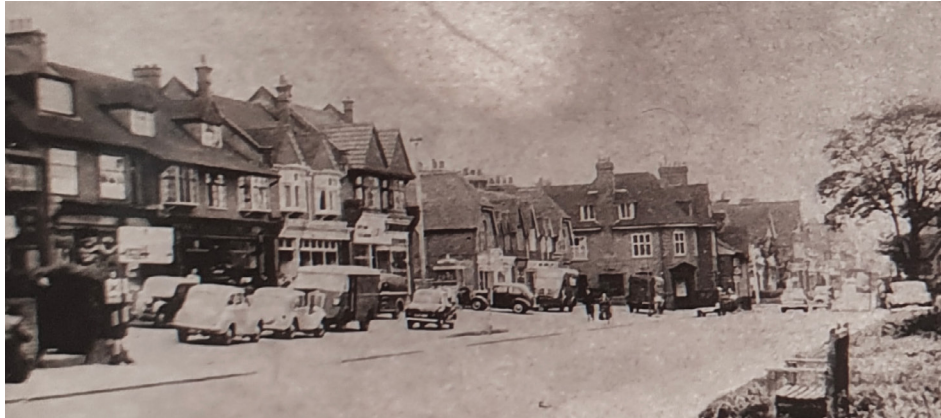
Fig 13. The Terrace in 1945. The parking apron is already in place but the east side of Watling Street is softened by a grassy verge and trees.
