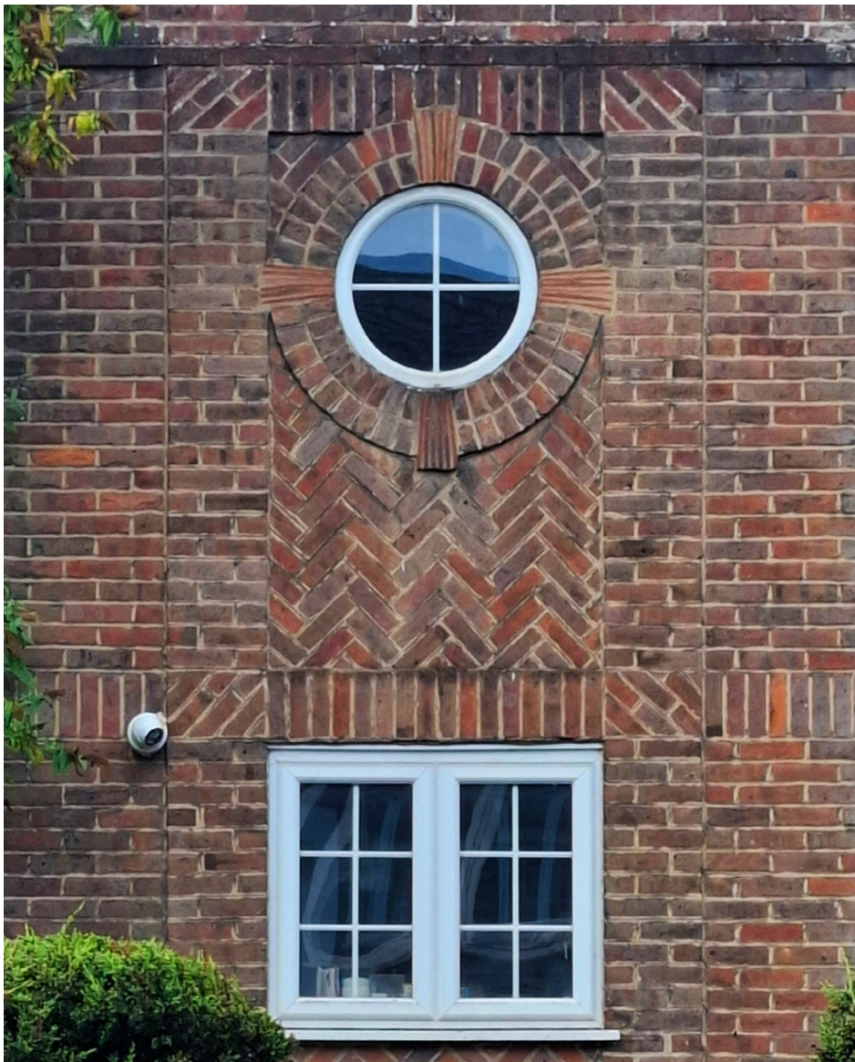
Fig 120. Red bricks with patterned detail
