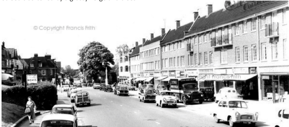
Fig 14. Watling Street in 1960. The grassy verge has gone and there is double parking on the wide pavement.
