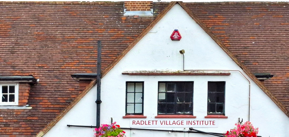
Fig 123. Gable and dormer
