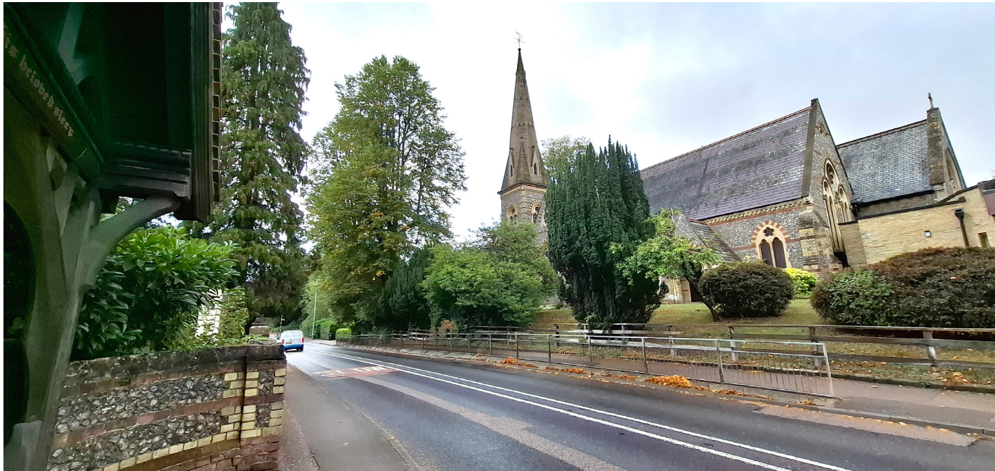
Fig 129. Views along Watling Street
